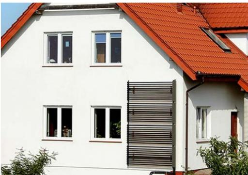
Also, the southern facade of the building may be used for the installation of solar collectors. In such a case, KS flat plate collectors use the KSOL universal constructions for the appropriate angle of inclination. KSR10 evacuated tube collectors can be installed in a vertical position and tubes can be turned by 25° to correct the unfavourable inclination of the absorbers.
